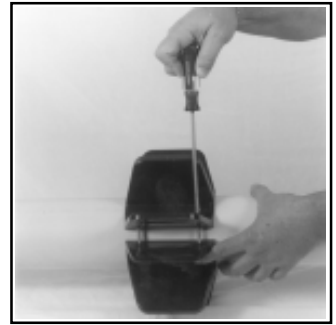
Place all sections around pipe and pull down allen bolts
